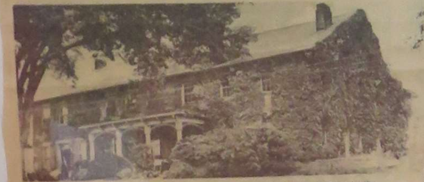
The Five Mile House near the entrance to Morchala Park was built for Cato James in 1830 and was used both as a
