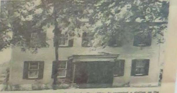
At the rear of this Stokely house one mile north of Roseville stands the older section in which Lydia Stokely operated a station on the Underground Railroad.
